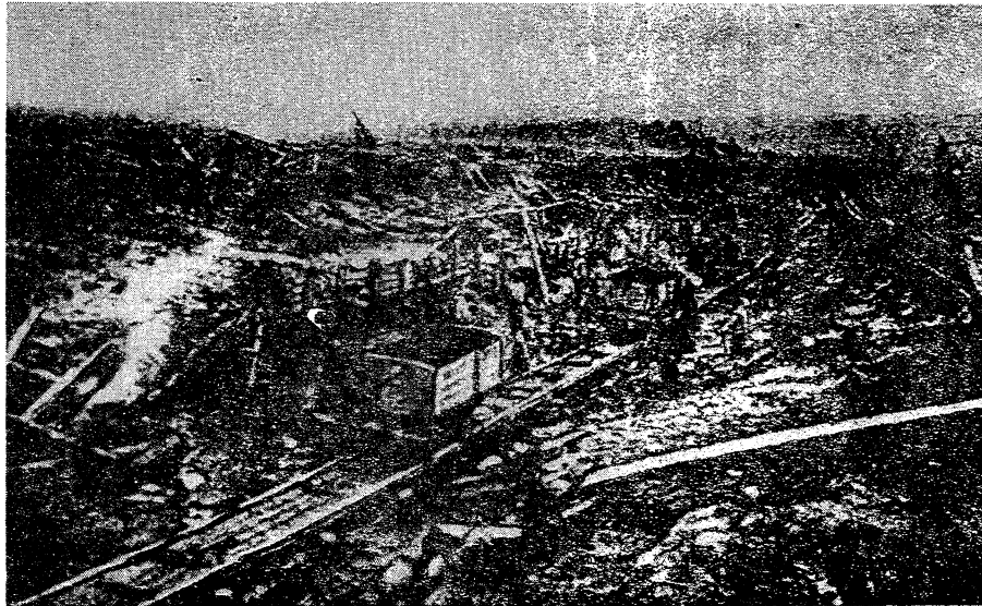
Fig. 152 - View of Excavation and Muddy Cut on the Amur Road
