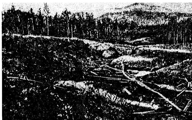
Fig. 63 - Cut Filled with Slud Due to Melting of Imbedded Ice
