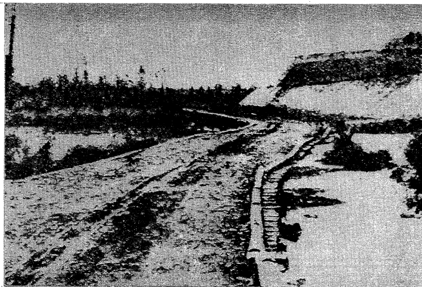
Fig. 136 - Temporary Road along the Amur Highway
