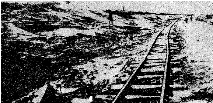
Fig. 150 - Muddy Cut with Sliding Slopes
