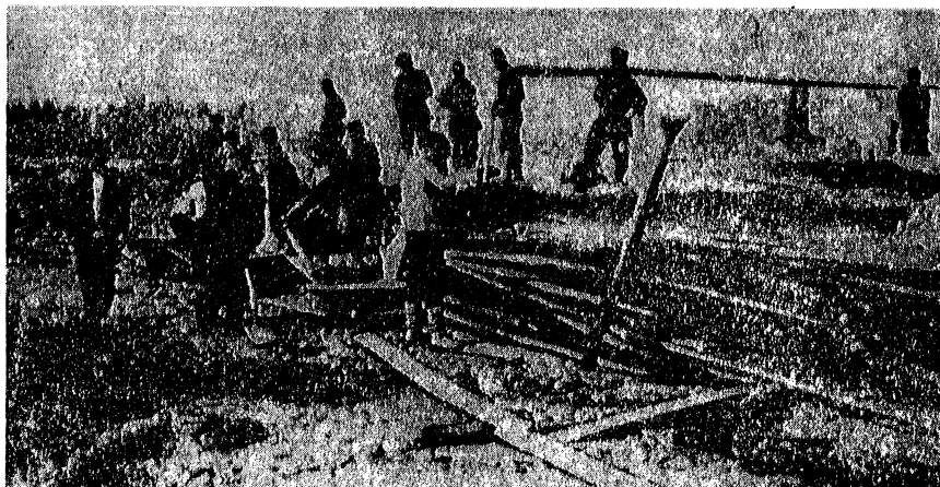
Fig. 153 - Thawing Operations with Bonfires
