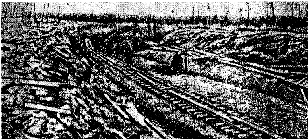
Fig. 62 - Muddy Railroad Cut During Construction
