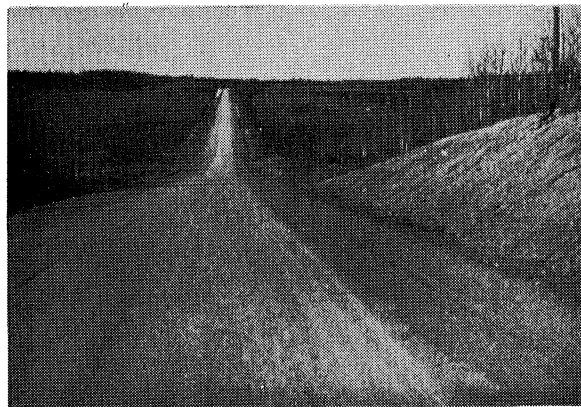
The cut slopes have been exposed to the weather for about four years without noticeable damage due to erosion.
