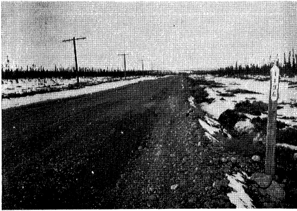
Settlement of the road grade was very uneven through this section which traversed flat terrain where the permafrost table was close to the ground surface. Alaska Highway in Western Yukon Territory
