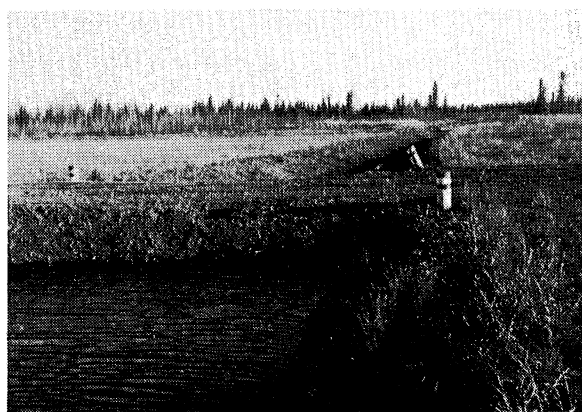
The culvert through this road grade was completely filled with ice.
