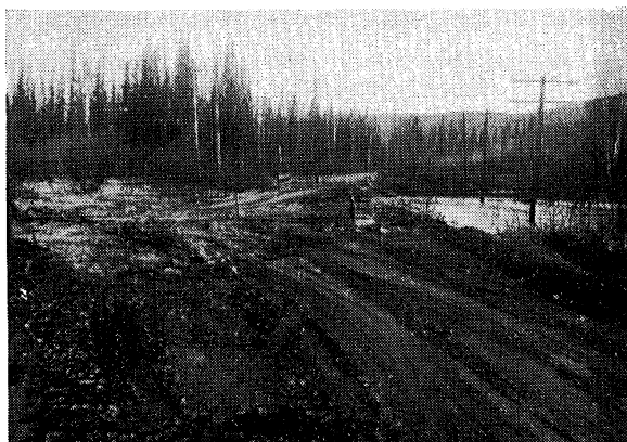
On May 15, 1949, high stages of Shaw Creek overtopped the highway and washed out a section of the grade.
