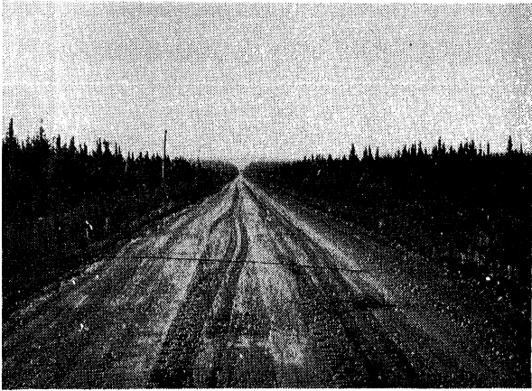
Road conditions are good despite a lack of drainage ditches.
