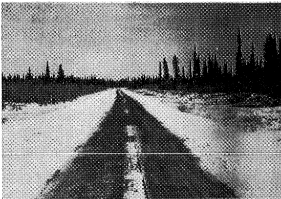
Burwash Creek Road at mile 1104. Many trees are in a tilted position.
