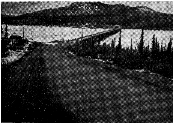
The longest wooden bridge on the highway crosses Nisutlin Bay of Teslin Lake.
