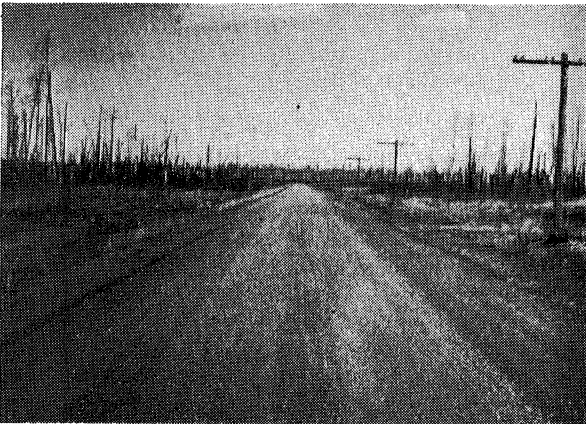
There are no side ditches to convey runoff.
