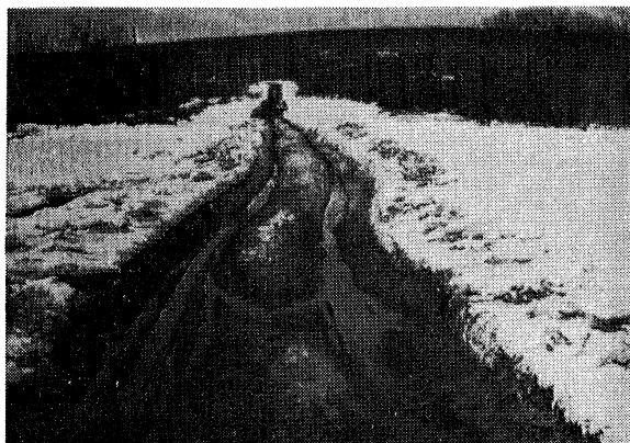
On May 6, 1949, the blasting operation of April 27 revealed the handrail of a culvert which had been completely covered with ice.
