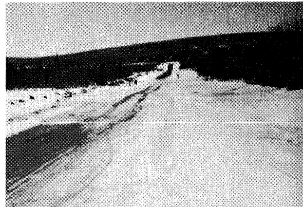
On April 27, 1949, highway maintenance men were drilling holes through the icing preparatory to a blasting operation to clear an outlet channel.
