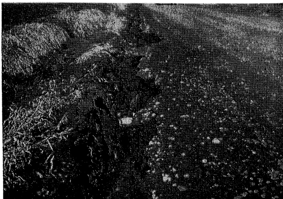
At both sites gullies had formed in a matter of a few days even though the active layer was still frozen.
