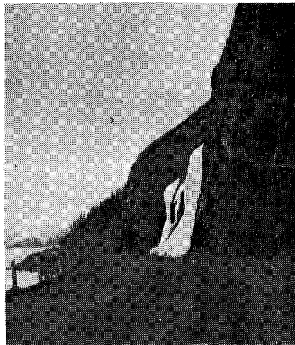
Water forming the icing comes from seepage through the fissures and crevices in the rock bluff.
