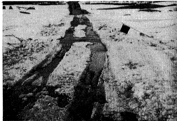
The bridge over Fox Creek was nearly filled with ice. This caused seepage through pervious tailings and overtopping of a low section of the road a short distance from the bridge.
