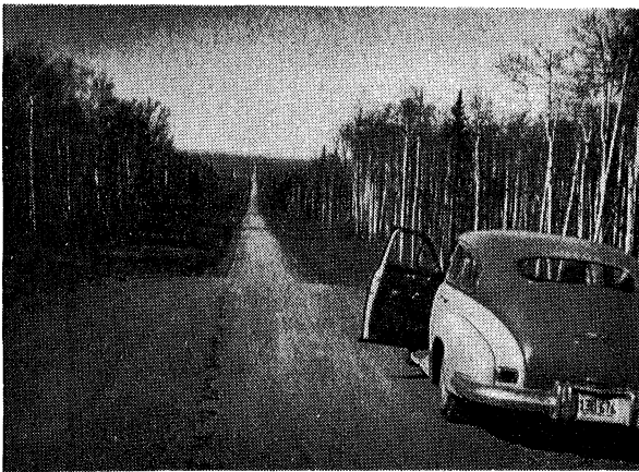
Road side ditches are conspicuously absent along this highway.
