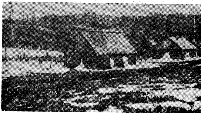
Water seeping through unfrozen ground beneath the house fills the building with ice.
