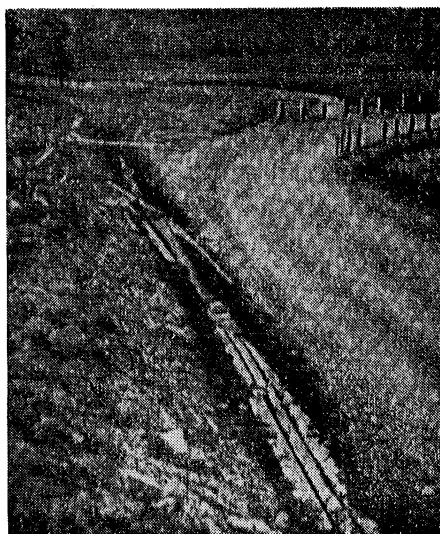
Fig. 32 - Insulated Ditch Covered During Winter, Amur-Yakutsk Highway
