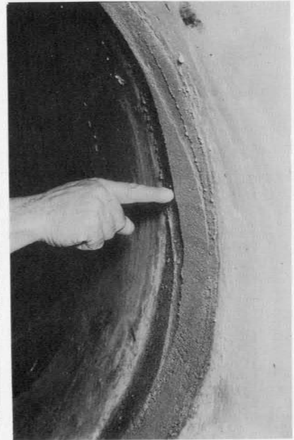
(c) Joint No. 23 in 36-in. cast pipe: 0.44-in. maximum offset plus 0.53-in. maximum bead height
