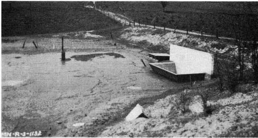
(a) Experimental 2 ft by 2 ft spillway has been capped and only headwall shows beyond twin 6 ft by 6 ft spillway.
