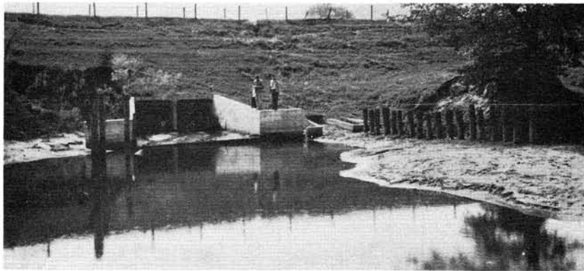
(b) Outlet has silted in.
