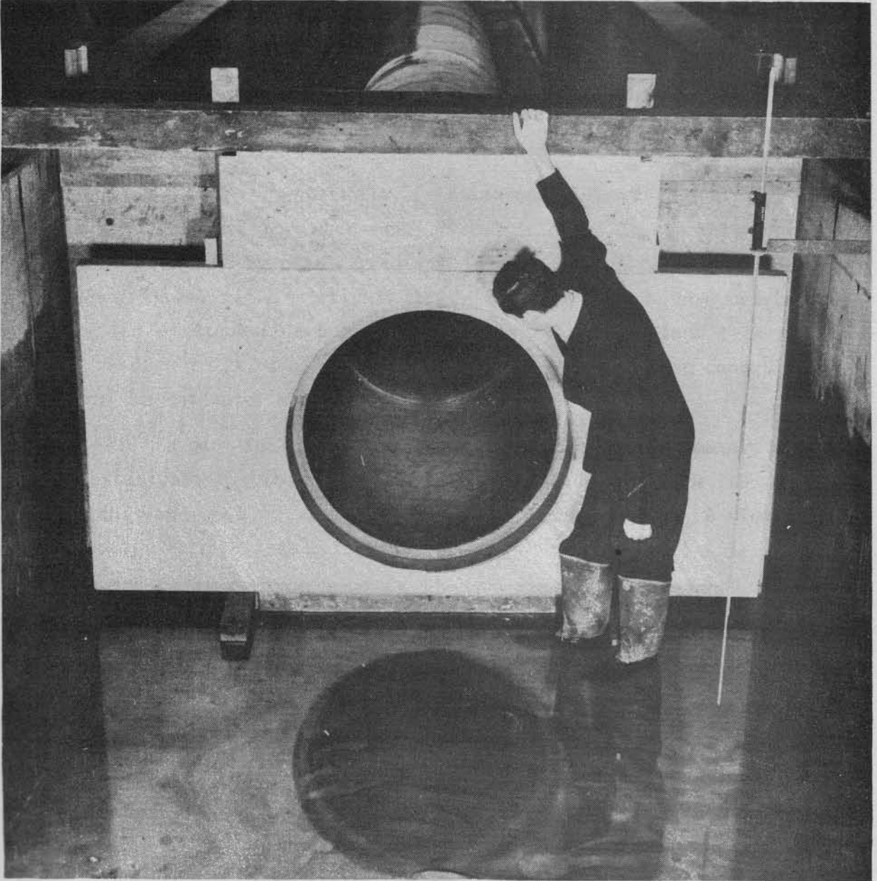
Fig. 2- Flush Headwall at Inlet to 36-in. Concrete Culvert
