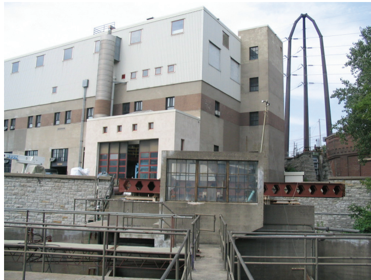
The SAFL building, as seen from the south side.
