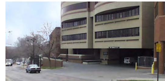
East River Road Service Docks
