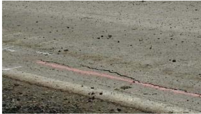
Figure 2.20. Failure at Cell 83 westbound lane on 18 March 2009
