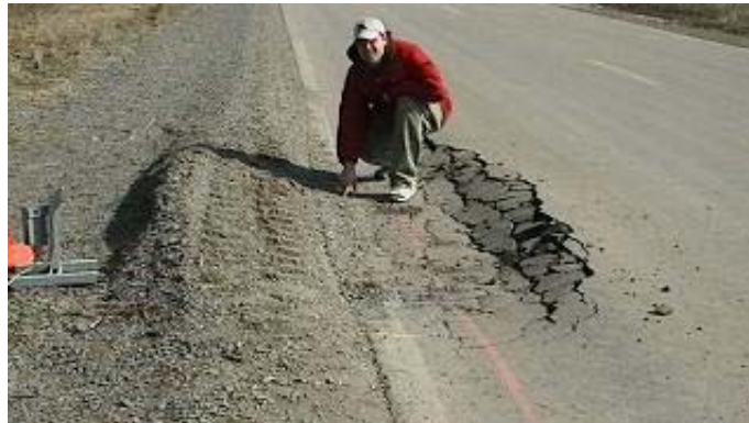
Figure 2.21. Failure at Cell 83 westbound lane on 19 March 2009
