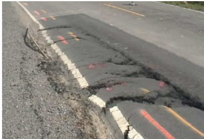
Figure 2.22. Slippage cracks at Cell 83 westbound lane on 24 August 2009
