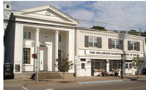
Figure 8, Façade, Delaware Bank
