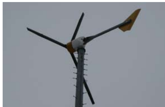
Figure 66: Wolf Ridge’s existing 10 kW wind generator
