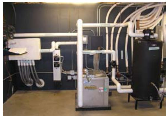
Figure 24: Utility Room, Biohaus
