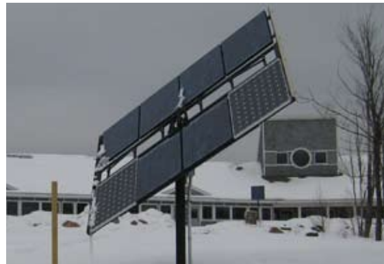
Figure 65: Wolf Ridge’s existing heliostatic 1 kW PV array
