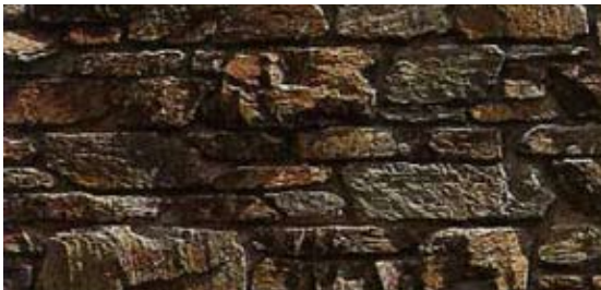
Figure 57: Detail, Residence, Ardennes
