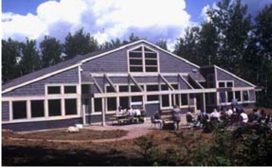
Figure 70: Forest Ecology Building, South Facade
