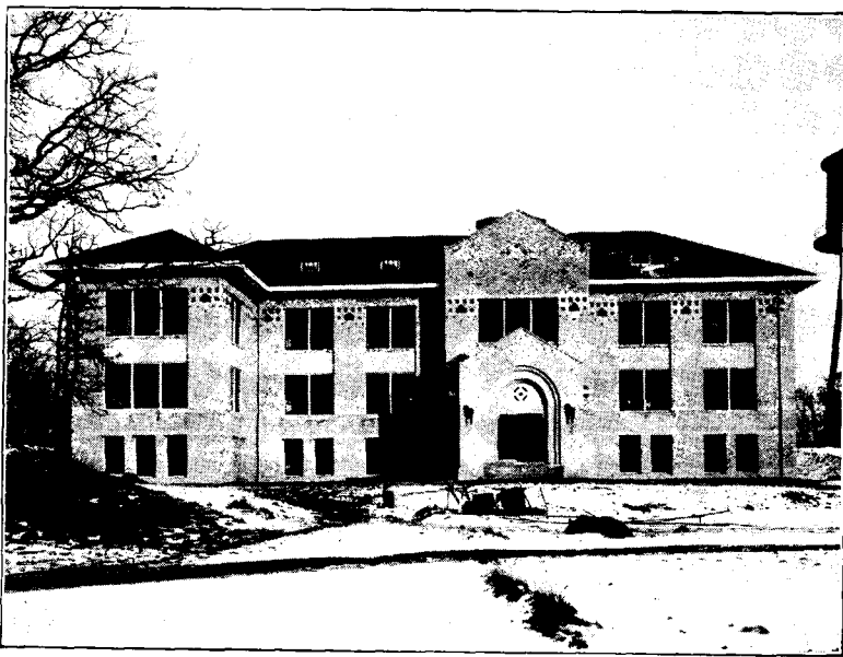
New Home Economics Building
