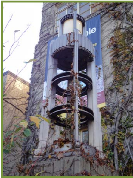
Figure 56: Bell Exterior Lighting Fixture
