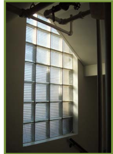
Figure 33: Decorative Glass Block Window in Stairwell
