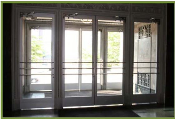
Figure 42: Frist Lobby Doors
