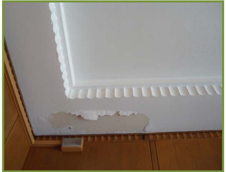
Figure 89: Water Damage on Vestibule Ceiling
