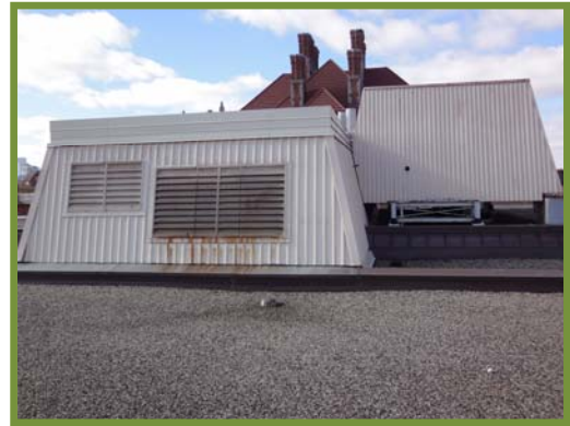
Figure 83: Addition's Air Handling Unit And Cooling Tower
