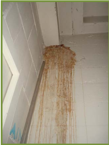
Figure 88: Water Damage In Stairwell
