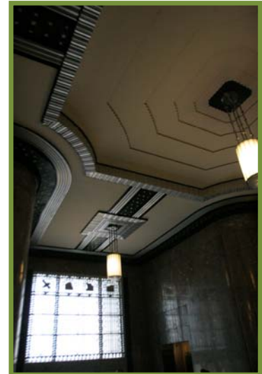
Figure 48: Frist Interior Ceiling Detail
