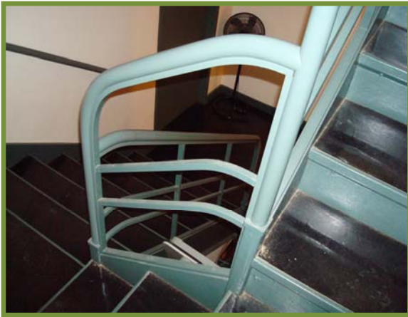
Figure 34: Back Stair Curved Metal Handrail
