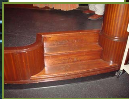
Figure 22: Auditorium Stage - Wood Stairs
