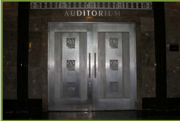
Figure 44: Interior Aluminum Doors with Marble Walls and Floors
