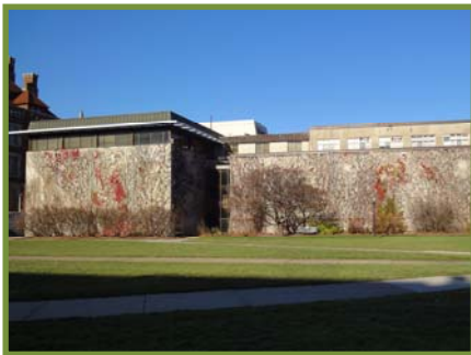
Figure 8: Southside of Bell Museum Showing Cooling Tower
