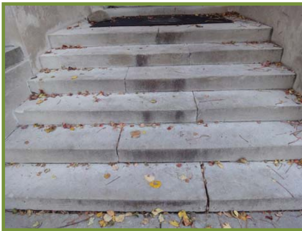
Figure 57: Bell Exterior Auditorium Stairs
