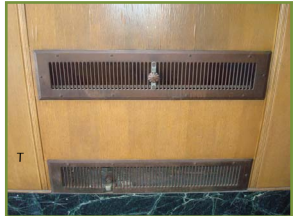
Figure 20: Vestibule Grillwork Hiding Radiators, and the Green Marble Wall Base
