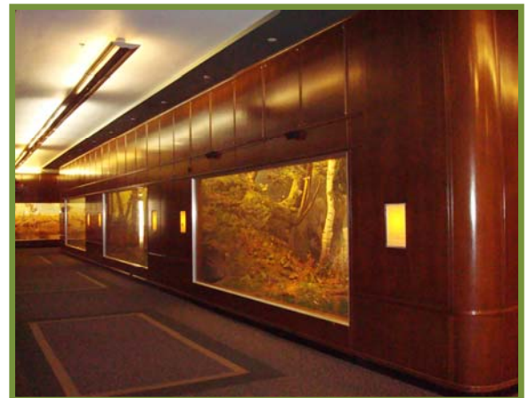
Figure 30: Rounded Paneled Wall Corner Per the Art Moderne /Art Deco Style.
