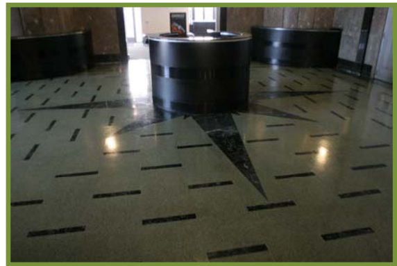
Figure 43: Frist Lobby Floor Pattern
