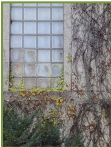
Figure 59: Bell Exterior Glass Block Window
