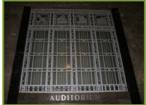
Figure 45: Interior Door Grillework
