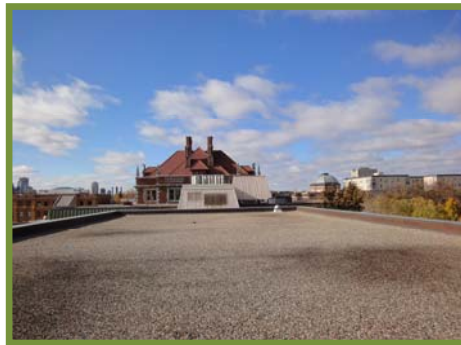
Figure 85: Main Roof Above Second Floor
