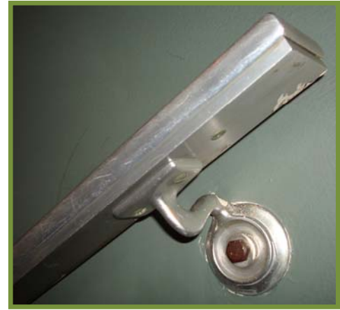
Figure 35: Curved Handrail Detail
