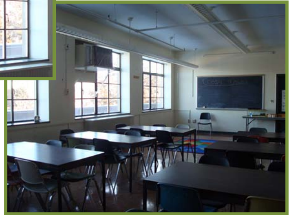
Figure 37A & B: Original Classroom Windows and Their Hardware
