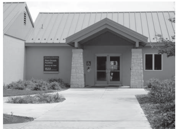
Entry into the renovated greenhouse facilities.
