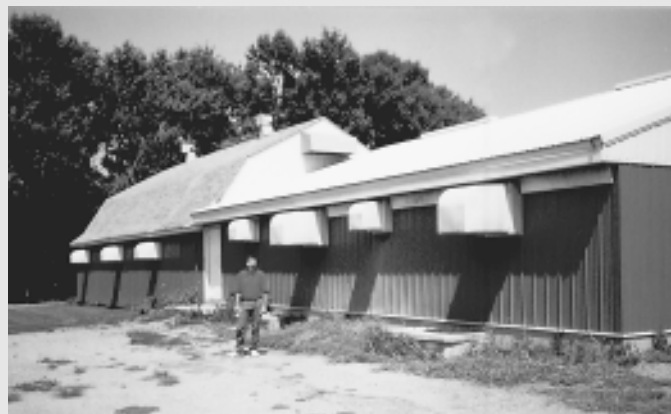
◆ Larry's barn remodeled for confinement operation.
