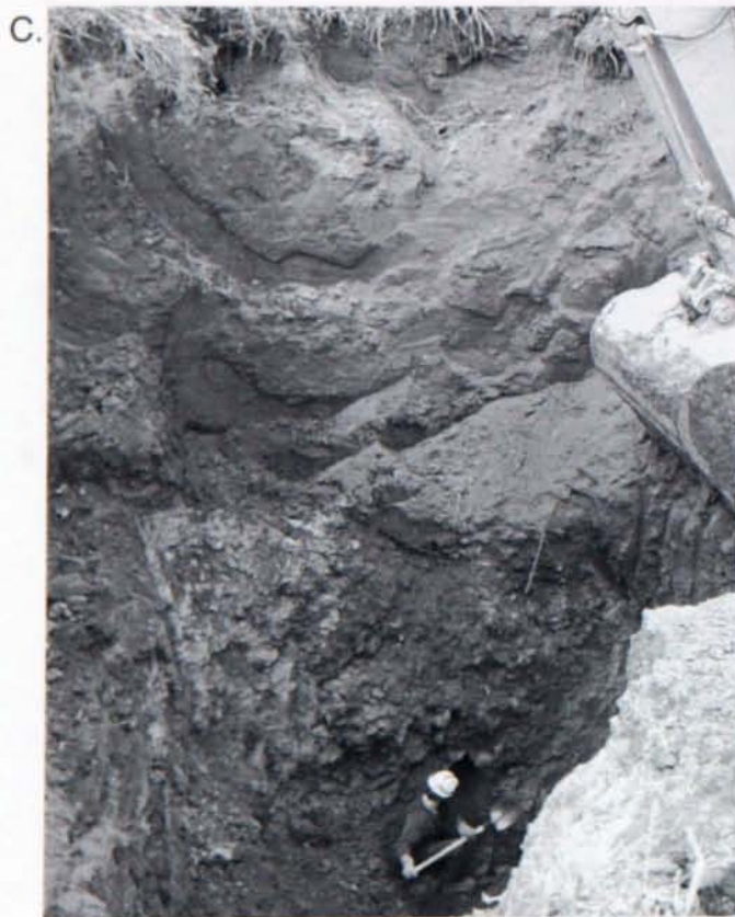
Figure 5.2. Sequence of photos showing the excavation of sinkhole MN23:D0074.
