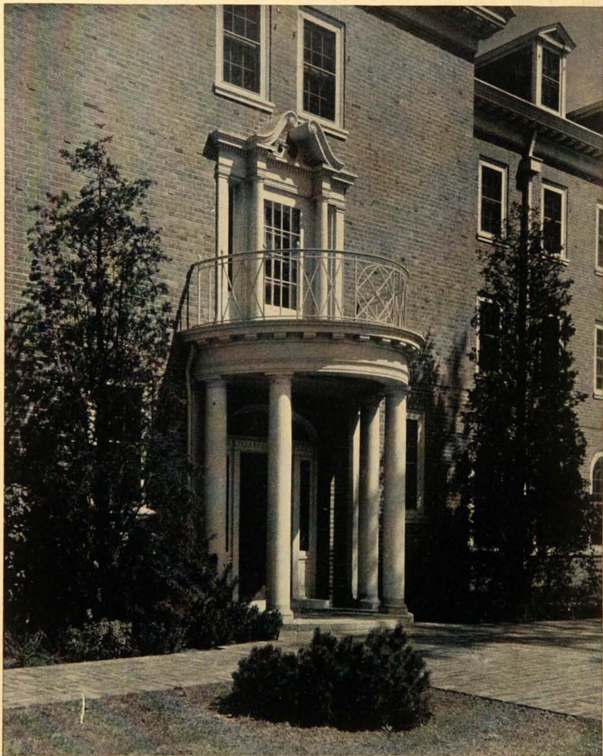
Main entrance to Pioneer Hall, residence for men students. Members of the Army and Navy training units at the University have been living in Pioneer Hall.
