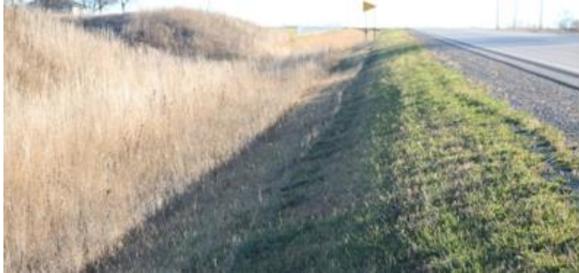
Figure 27: Steep backslopes at the Lac Qui Parle County site
