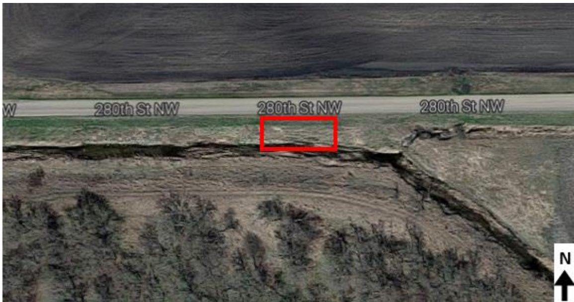
Figure A7.2: Marshall County site image
