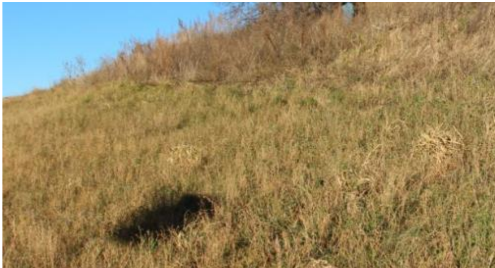
Figure 4: Naturally vegetated slope in Lac Qui Parle Co., MN
