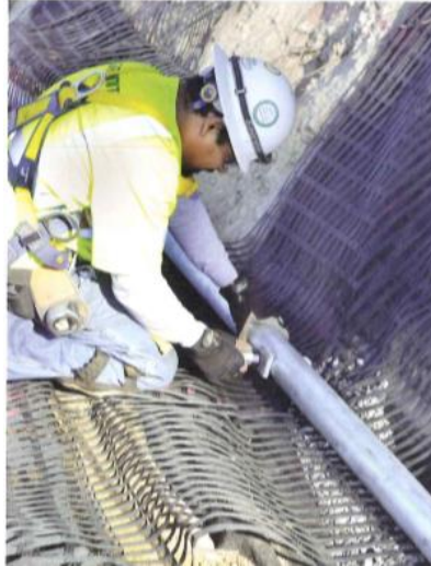
Figure 12: A worker anchors geogrid at the Lake Tahoe project (from Westfall, 2014)
