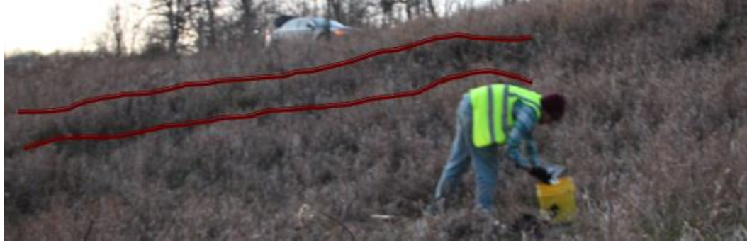
Figure 22: Clear rotational failure visible behind researcher at Fillmore County site
