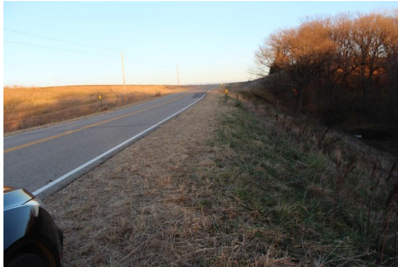
Figure 30: Murray County site slope after reconstruction with visible pavement repair
