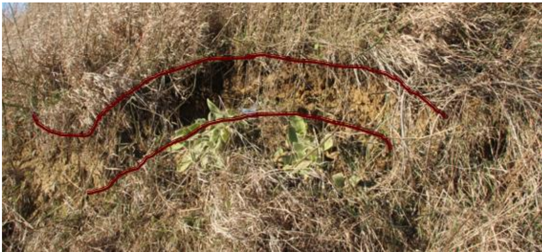
Figure 32: Rotational failure scarp at Olmsted Co. site
