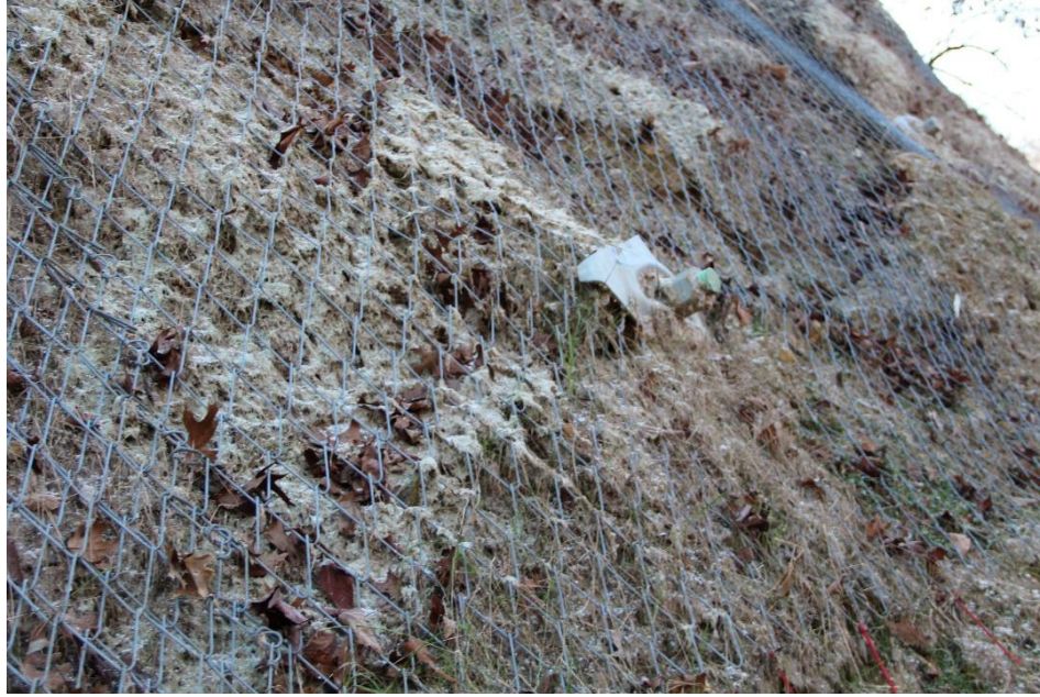
Figure 11: Rock bolts in combination with mesh cover in Washington Co., MN
