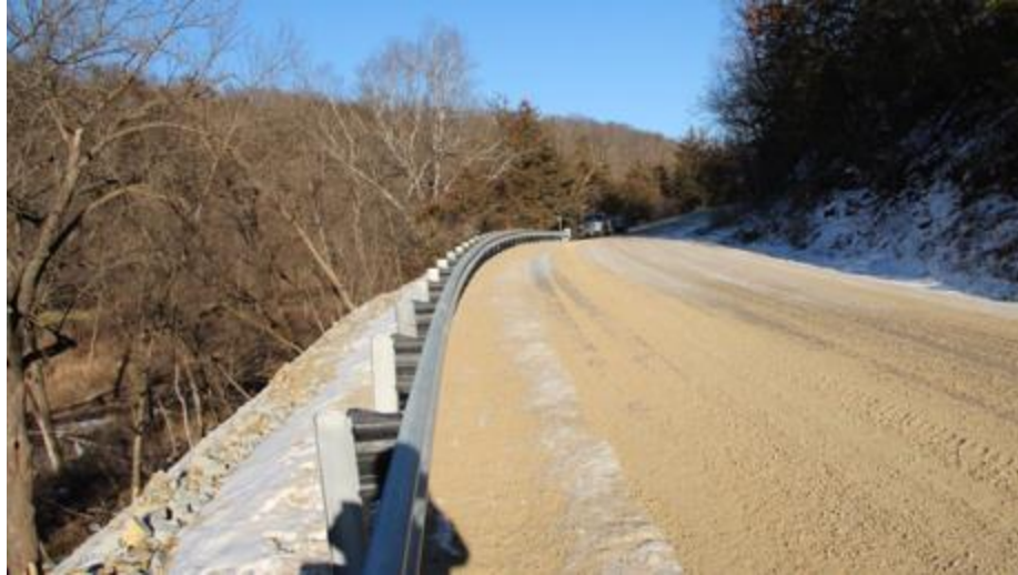
Figure 25: CSAH 19 (Houston County site) with steep uphill and downhill embankments
