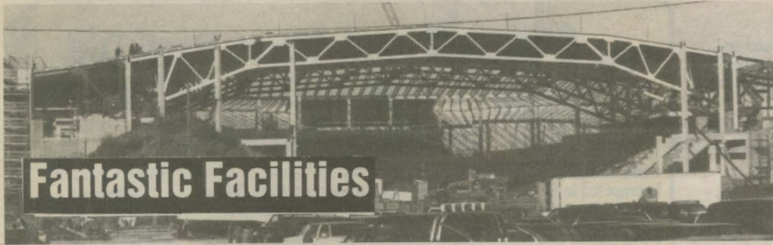
Left: Construction of new Mariucci Hockey Arena
